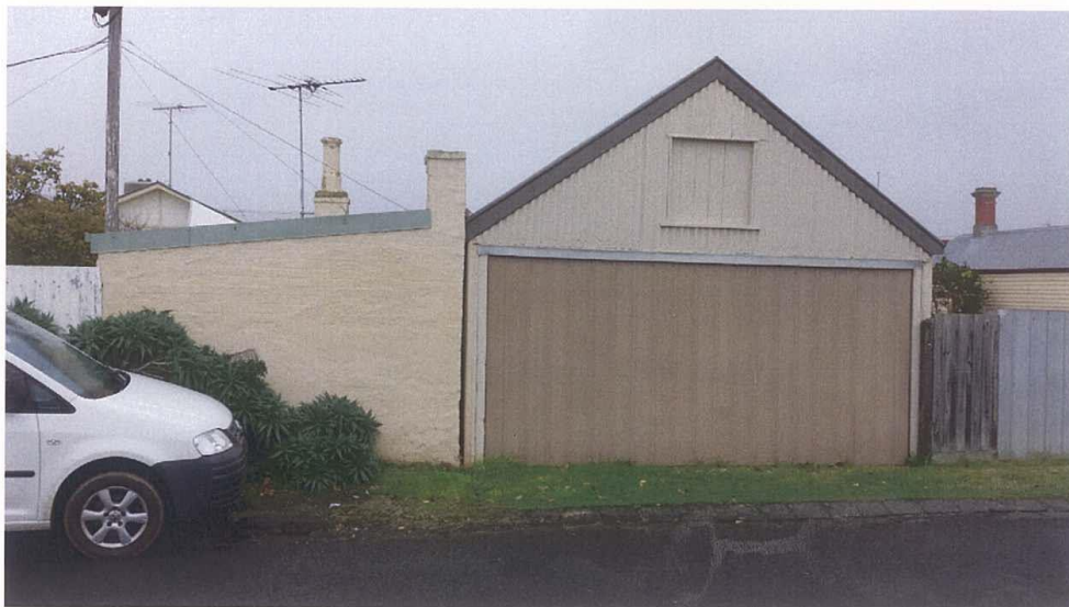
VIEW OF EAST WALL OF OUTBUILDINGS AT 12 KING STREET (GARAGE SHOWN IS TO BE DEMOLISHED)
