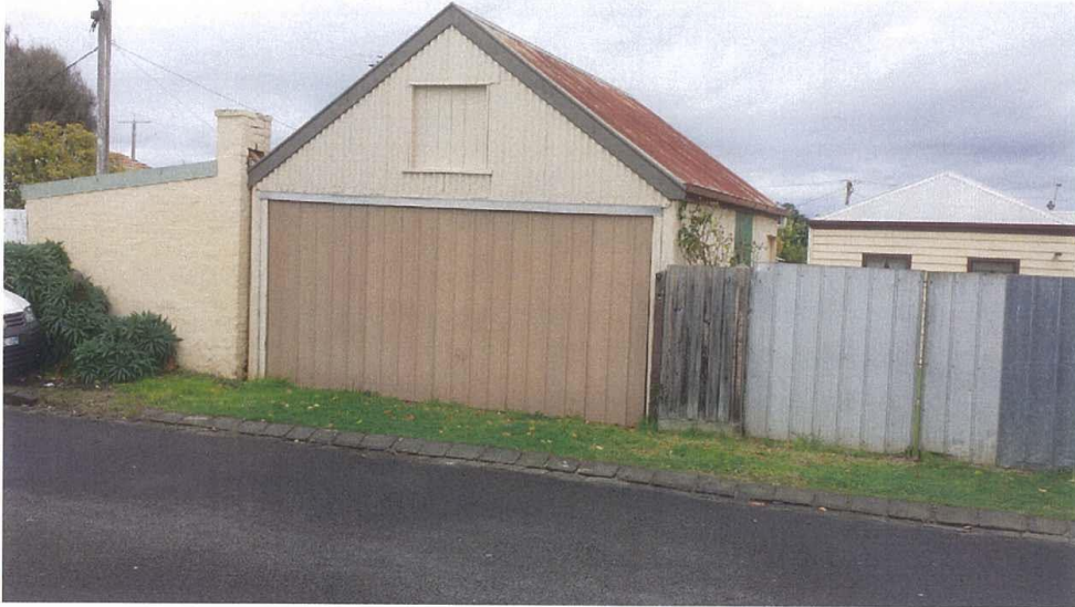
VIEW OF EXISTING GARAGE AND FENCING TO BE DEMOLISHED AND REPLACED
