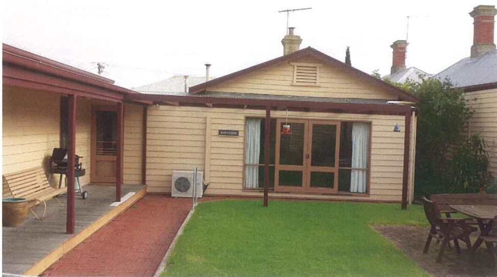
REAR OF EXISTING BUILDING SHOWING GRASSED AND PAVED AREA TO HAVE NEW LOW LEVEL DECKING INSTALLED OVER
