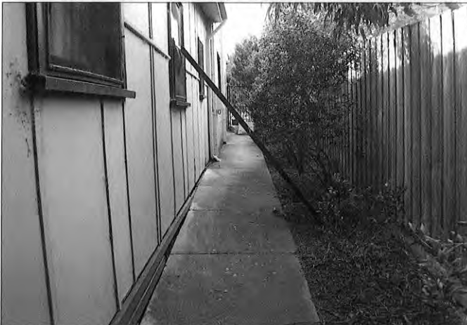
Southern side of the demolished dwelling.
