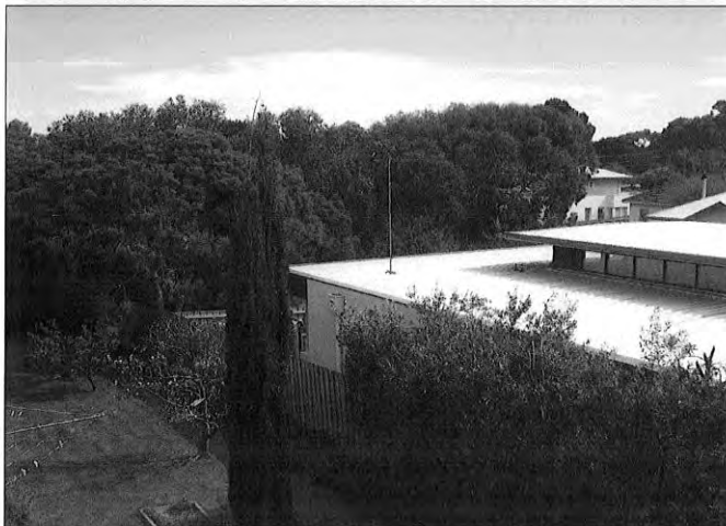
View to dwelling at 6 Arkins Street from previous rear first floor deck.
