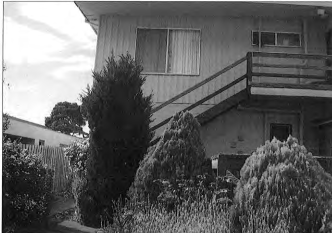
Rear section of the demolished dwelling.
