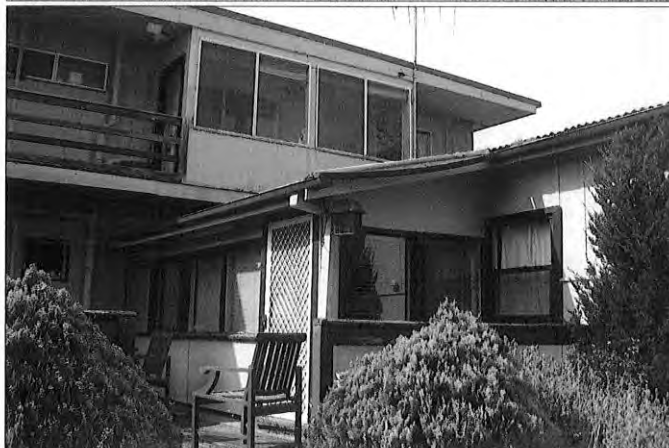
Rear section of the demolished dwelling.
